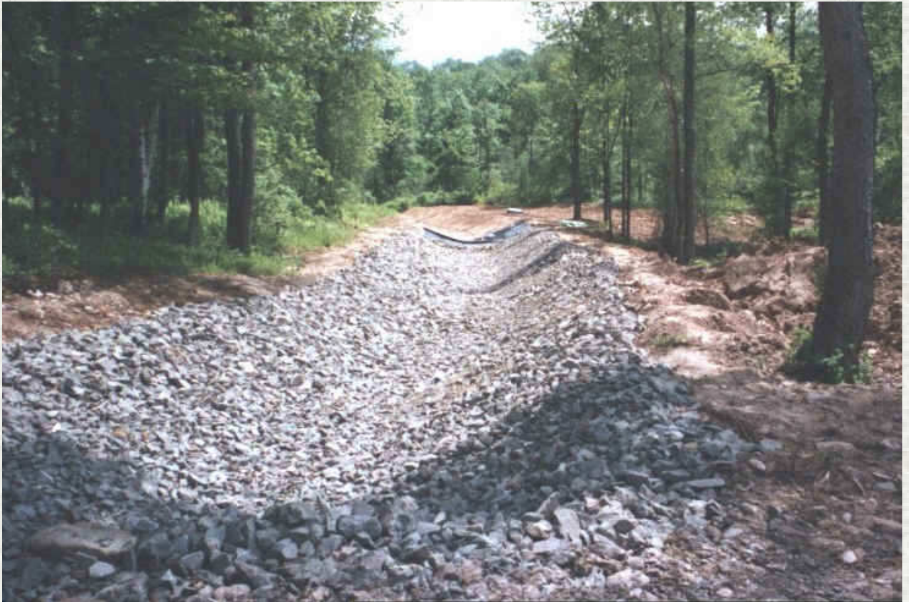
LIMESTONE DIVERSION CHANNEL
