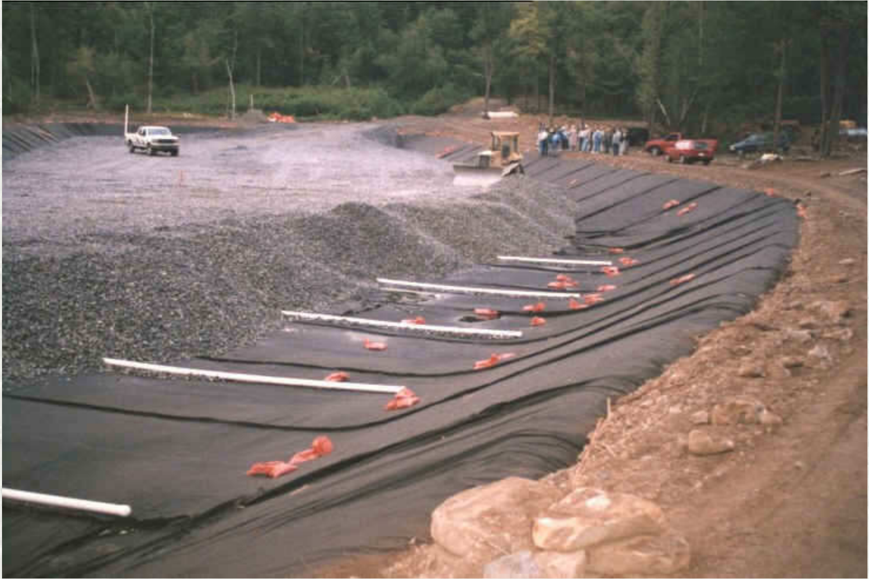
LIMESTONE AGGREGATE PLACEMENT IN POND
