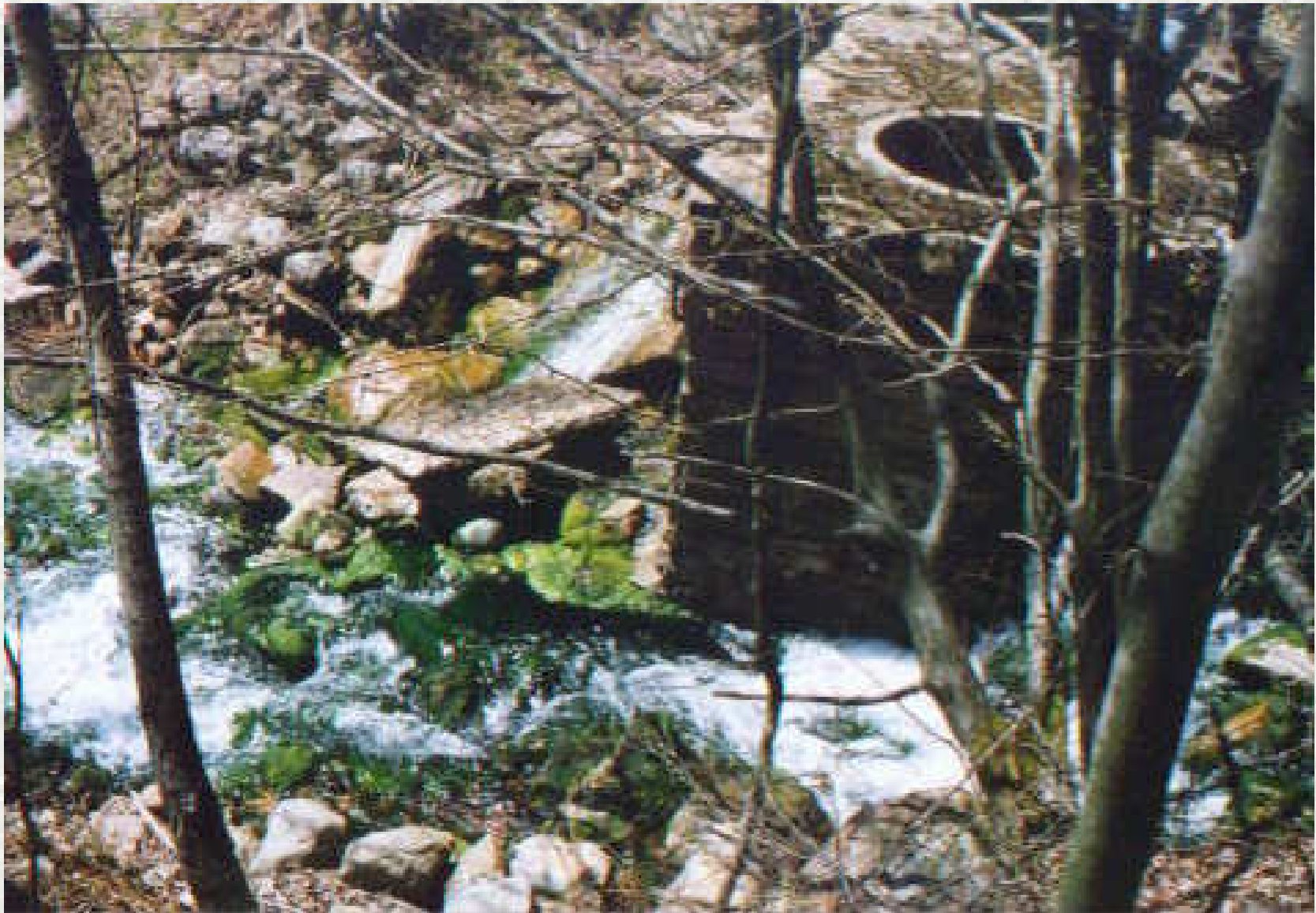
MINE DISCHARGE TUNNEL SOUTH OF LOPEZ
