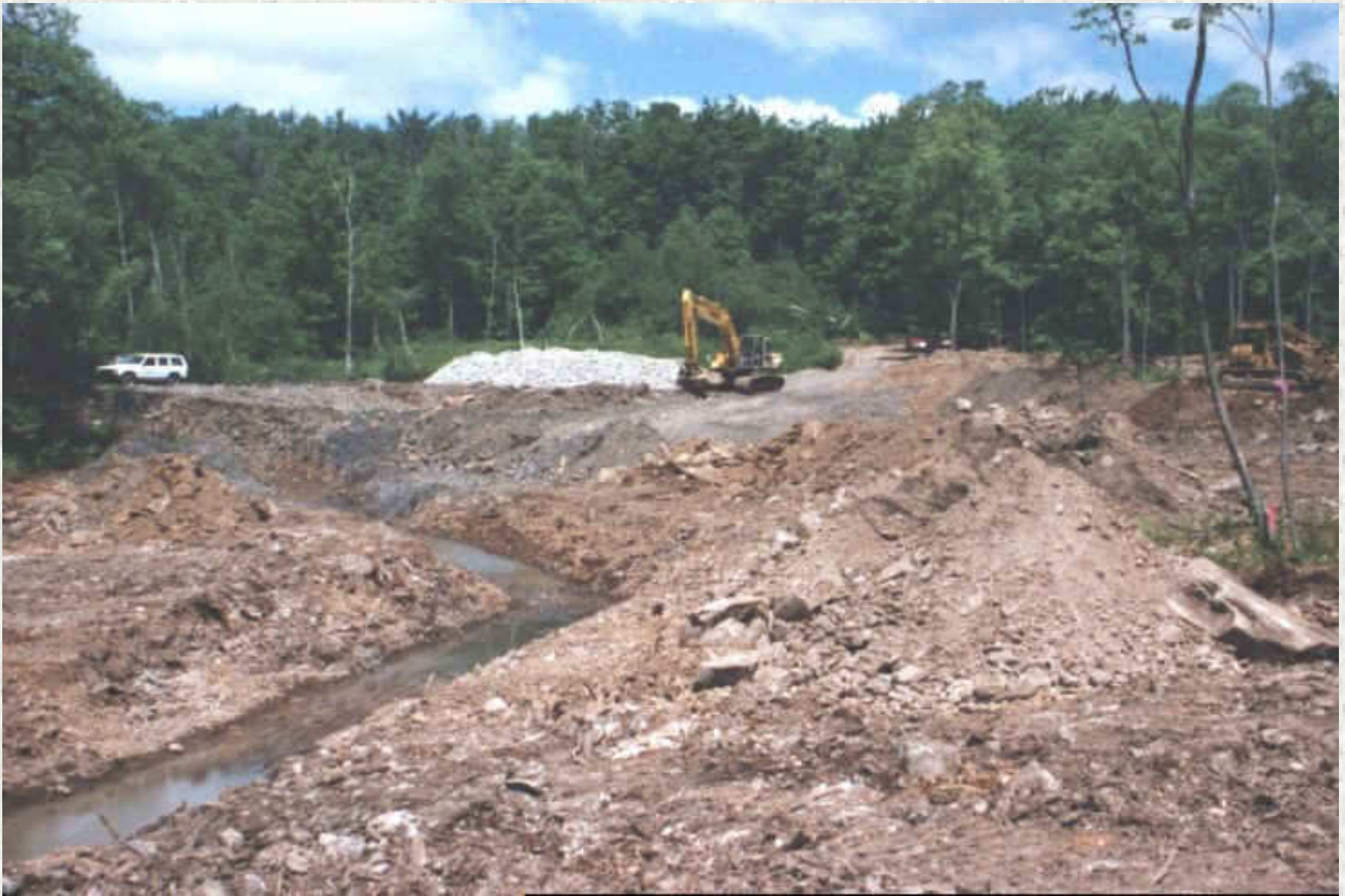
DIVERSION OF ACIDIC WATER DURING CONSTRUCTION
