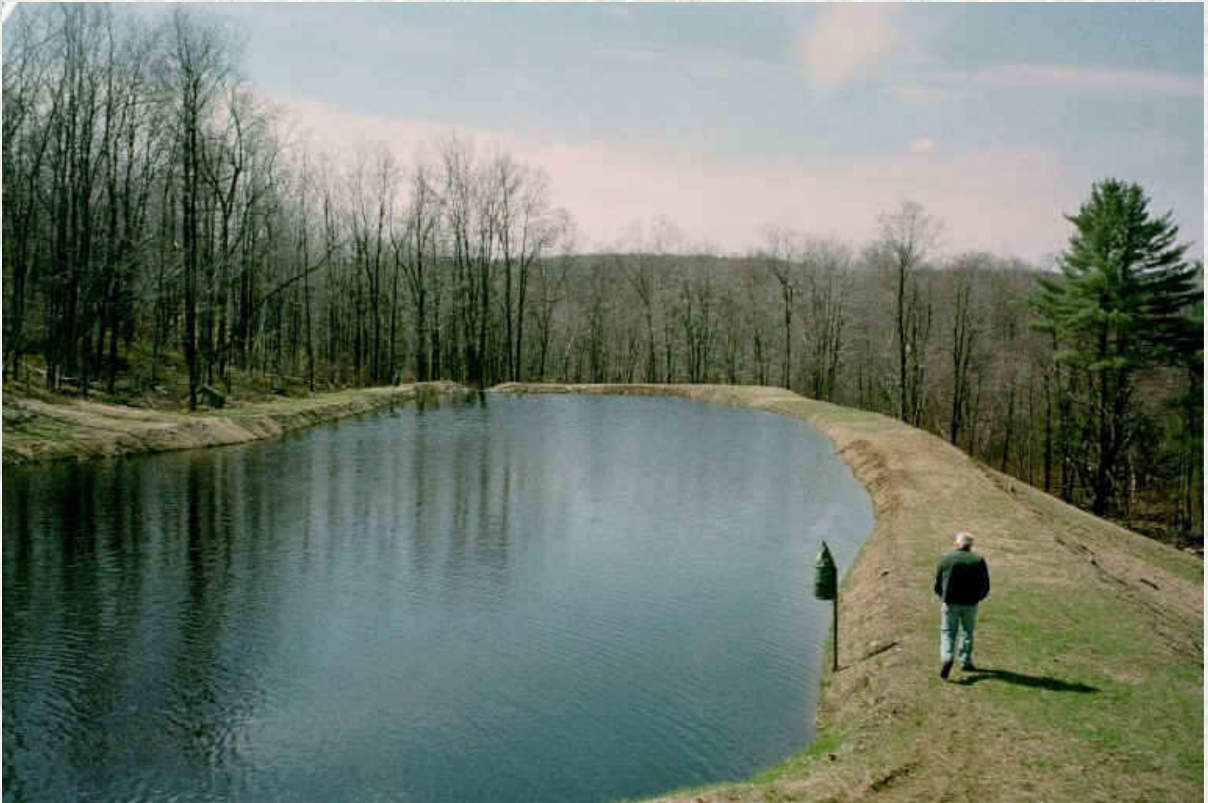
COMPLETED SETTLING POND
