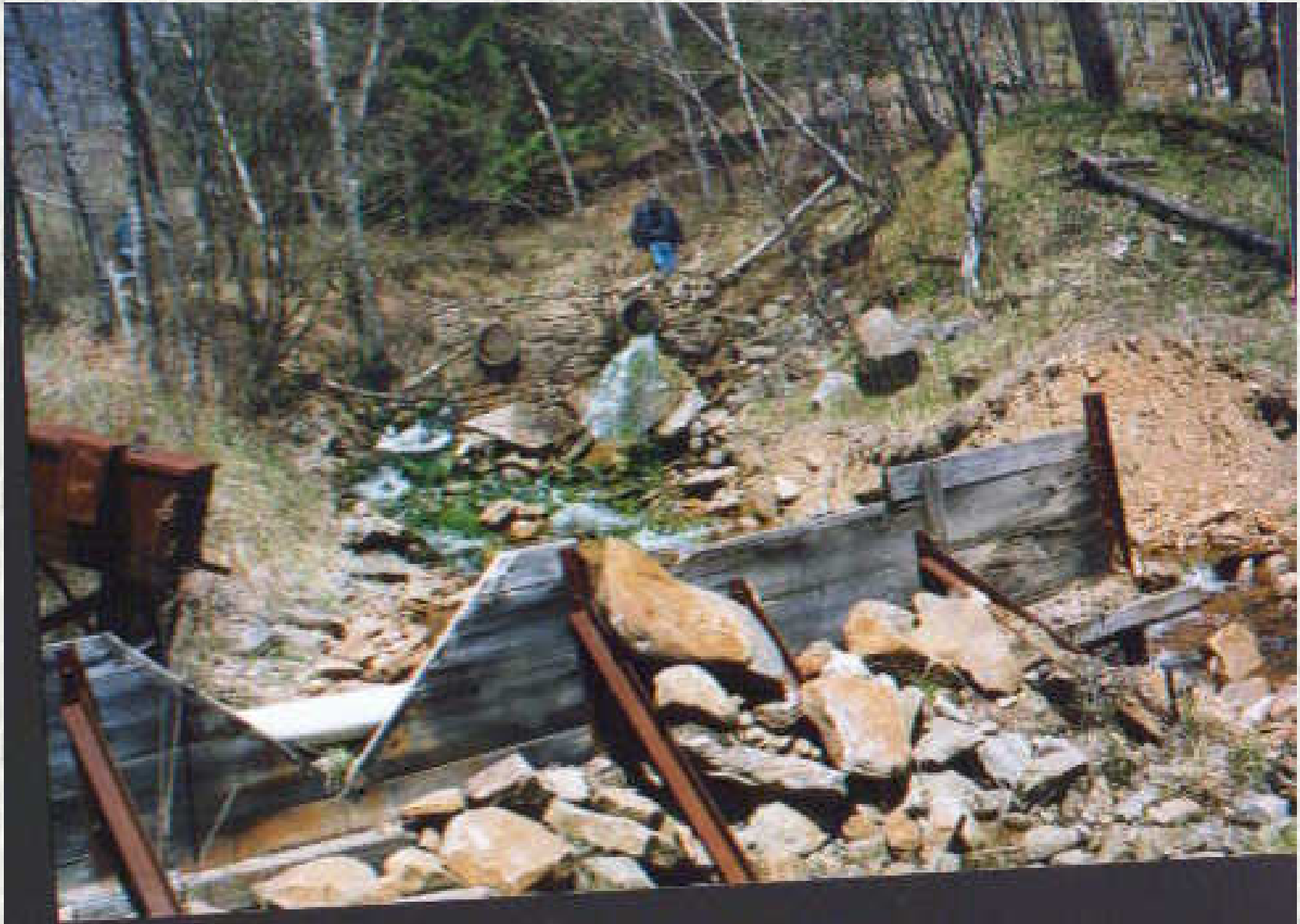
MINE DISCHARGE WITH REMINENTS OF PAST TESTING
