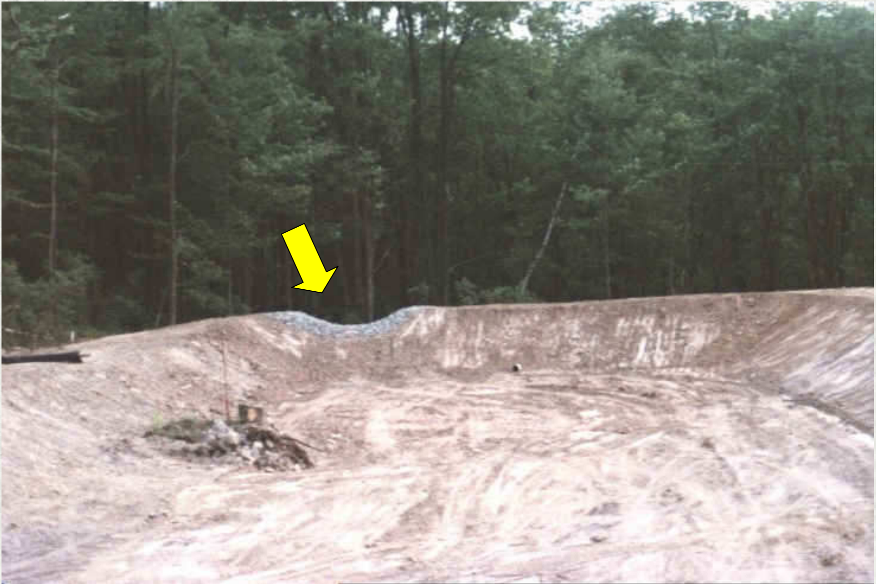
OUTFALL SETTLING POND TREATED WATER EXITS AT ARROW
