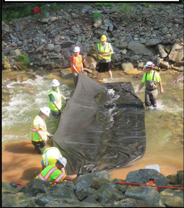
Geofabric installation on a cross vane structure on Hoagland Branch
