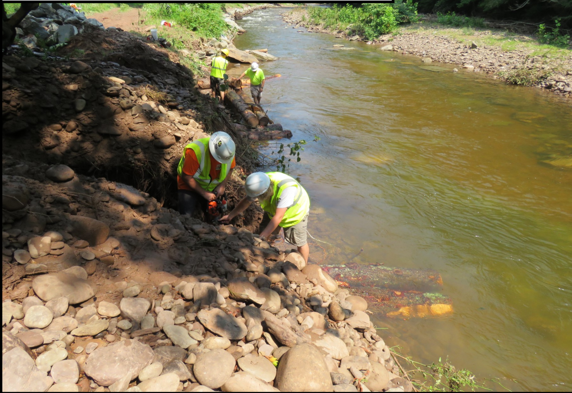
Construction of multi-log trout habitat structures on Elk Creek
